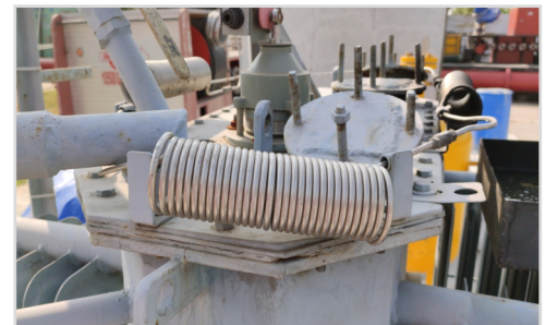
HEAT DETECTION TUBE ON A TRANSFORMER
