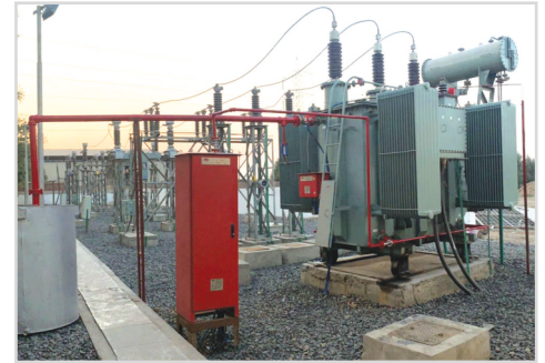
NITROGEN INJECTION SUPPRESSION UNIT
